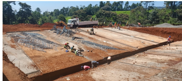
Ongoing construction of the sedimentation tank for Chogoria Water Supply
