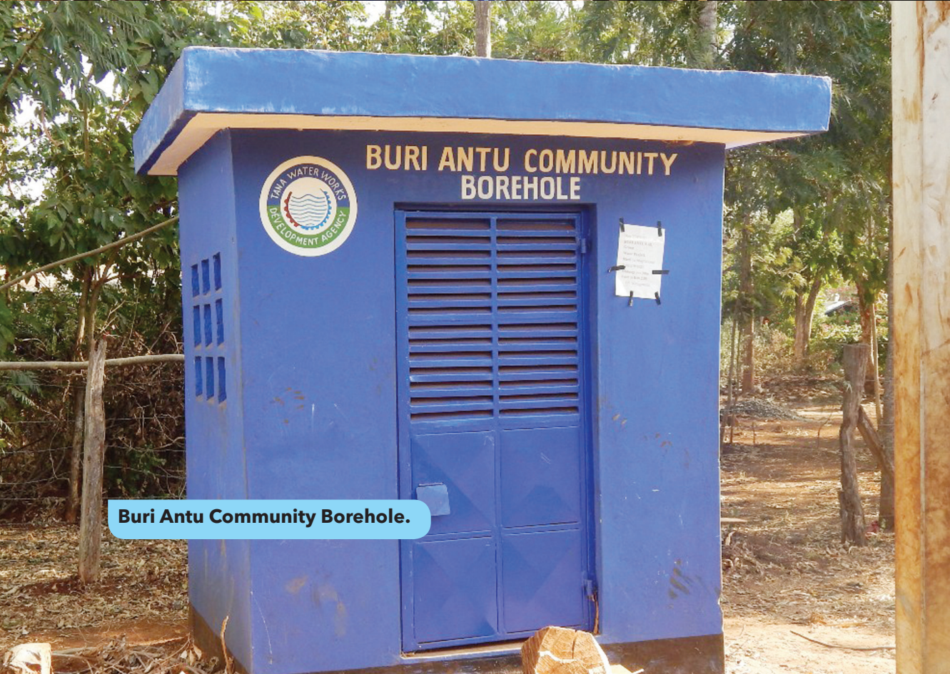
Buri Antu Community Borehole Solar-panels, Meru County.
