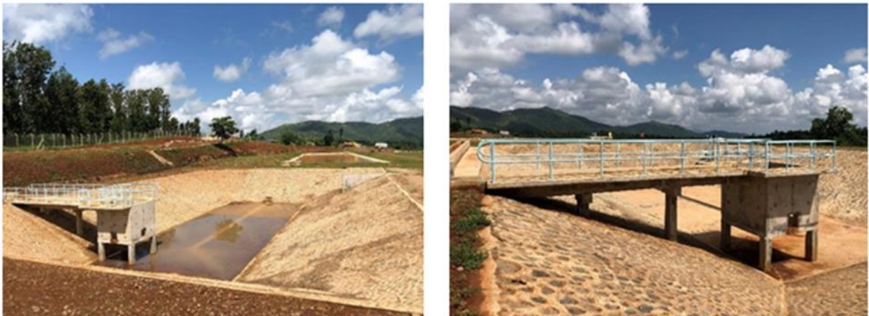
Figure 3.3: Anaerobic Pond
