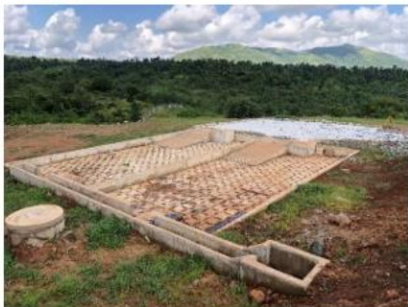
Figure 3.6: Sludge Drying Beds
