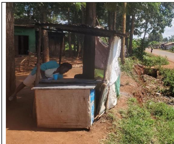
Figure 14: Grocery kiosk along the wayleave that would be demolished to pave way for excavation
