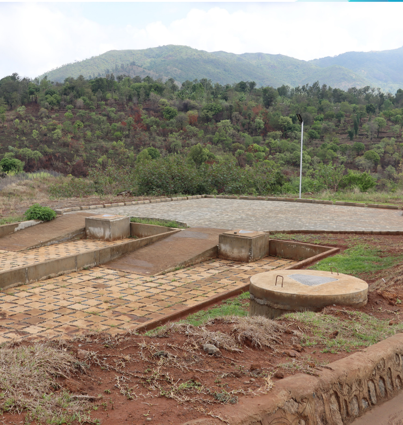
Chogoria SEwerage - Sludge Drying Beds
