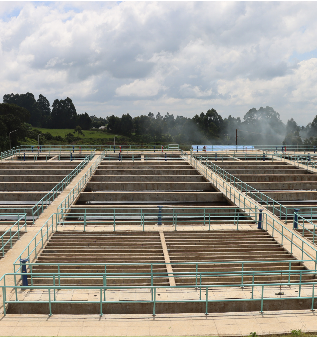
Kerugoya Kutus Water Treatment Plant
