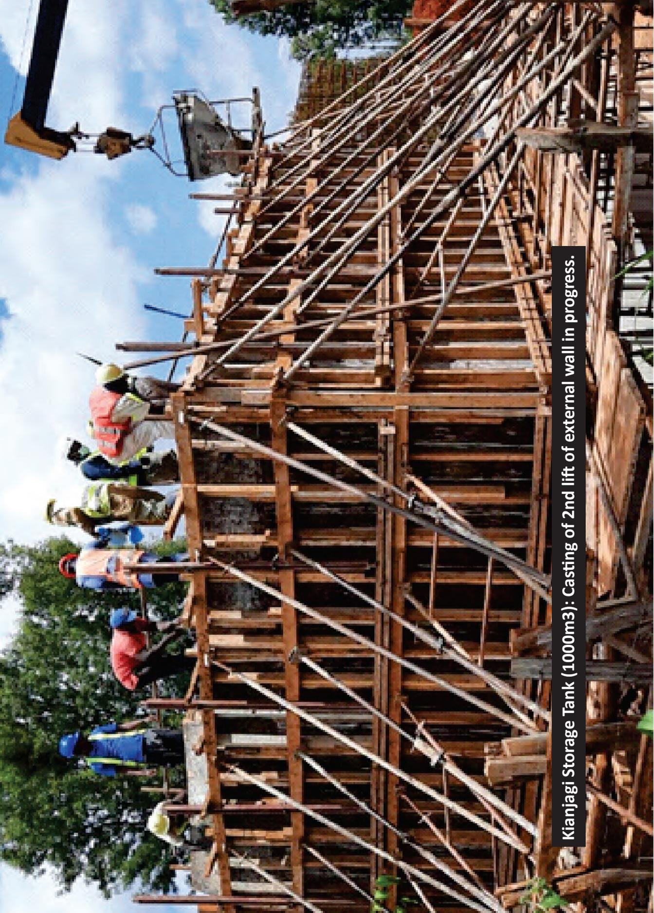
**Kianjagi Storage Tank (1000m3): Casting of 2nd lift of external wall in progress.**
