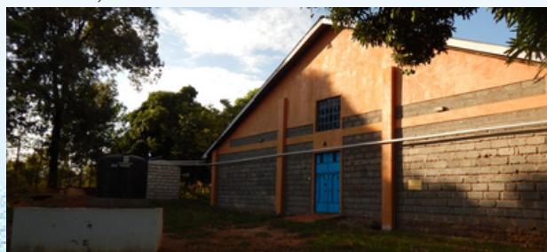
Rain Water Harvesting from A.C.K St. Barnabas Secondary School Kavengero Dining Hall
