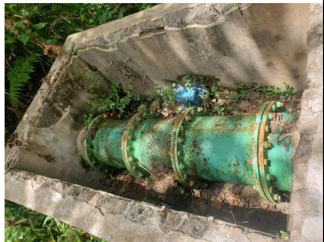
Wash out chamber for other projects within the forest ecosystem
