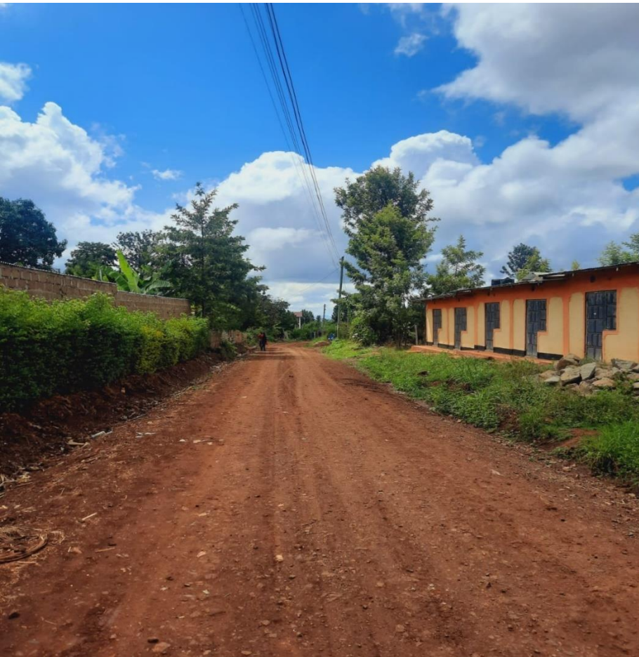
Figure 2-4: A section of road reserve to be utilized by the sewer line in Kiringani, Chuka
