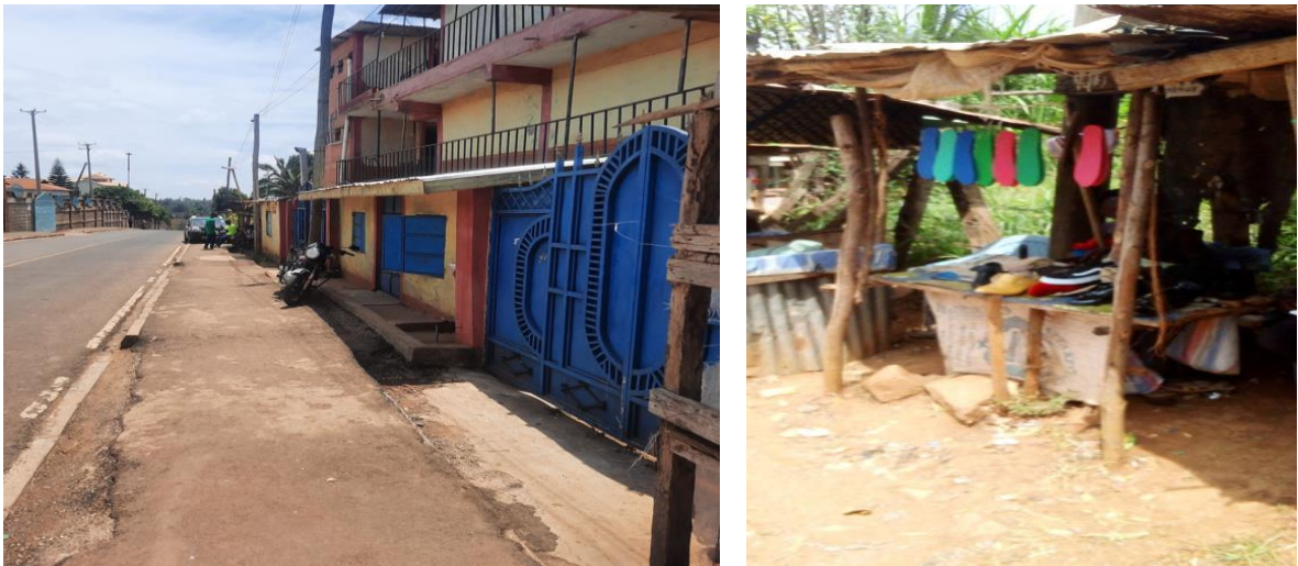
Figure 5-2: A concrete pavement and a temporary business structure to be affected by the project in Chuka town
