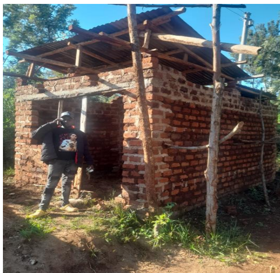
Figure 5.1: House under construction
